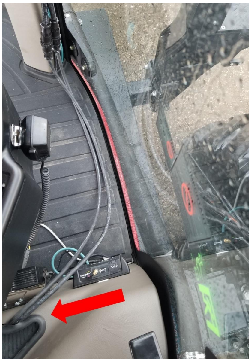
Fig. 13: Power Cables Routed Into Cab (Case IH Patriot)
